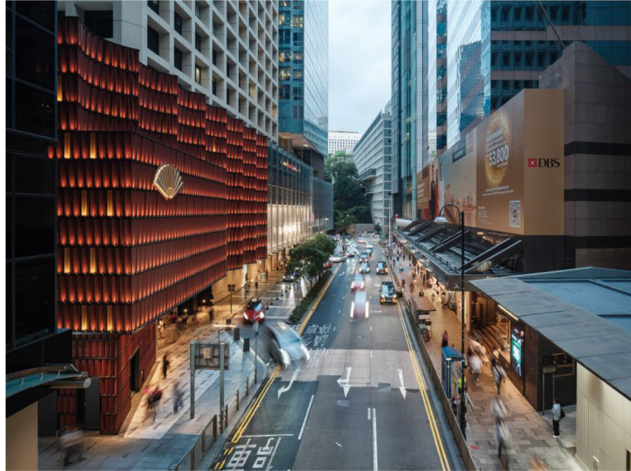
The newly renovated hotel is located at Hong Kong's Central district
