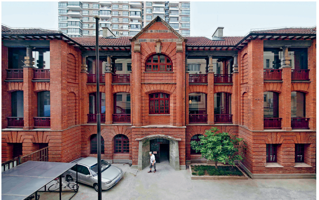
Above: Design Republic (2012), in central Shanghai, repurposes the former British police headquarters built in the 1910s. Nerù&flu adopts a surgical approach to the renovation, selectively removing floor slabs, walls, and ceiling panels to reveal the original structure, restoring the red brick masonry, and inserting new glazed volumes and contemporary interiors. Crisp white spaces are juxtaposed with raw surfaces, deteriorated plaster, and exposed timber laths
